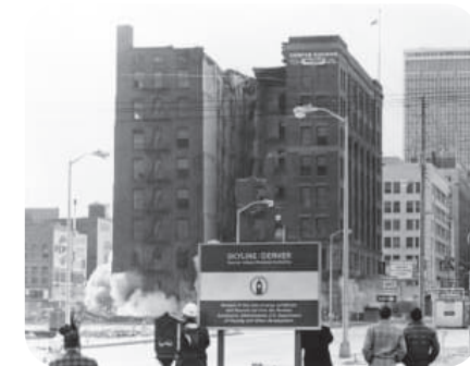
Skyline Urban Renewal-Cooper Building Demolition, 1970
