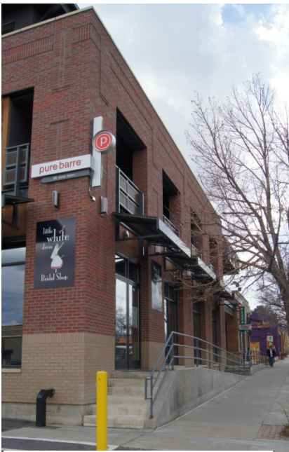
A building with a raised ground floor that required steps and a ramp to provide access to the building entrance.
